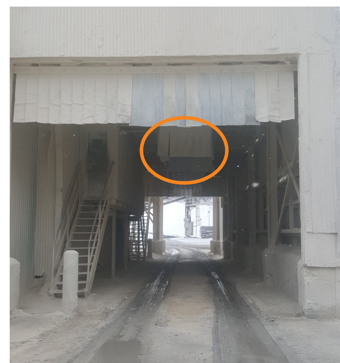
February 2021: Bin 12/13 Loadout area dust curtains
