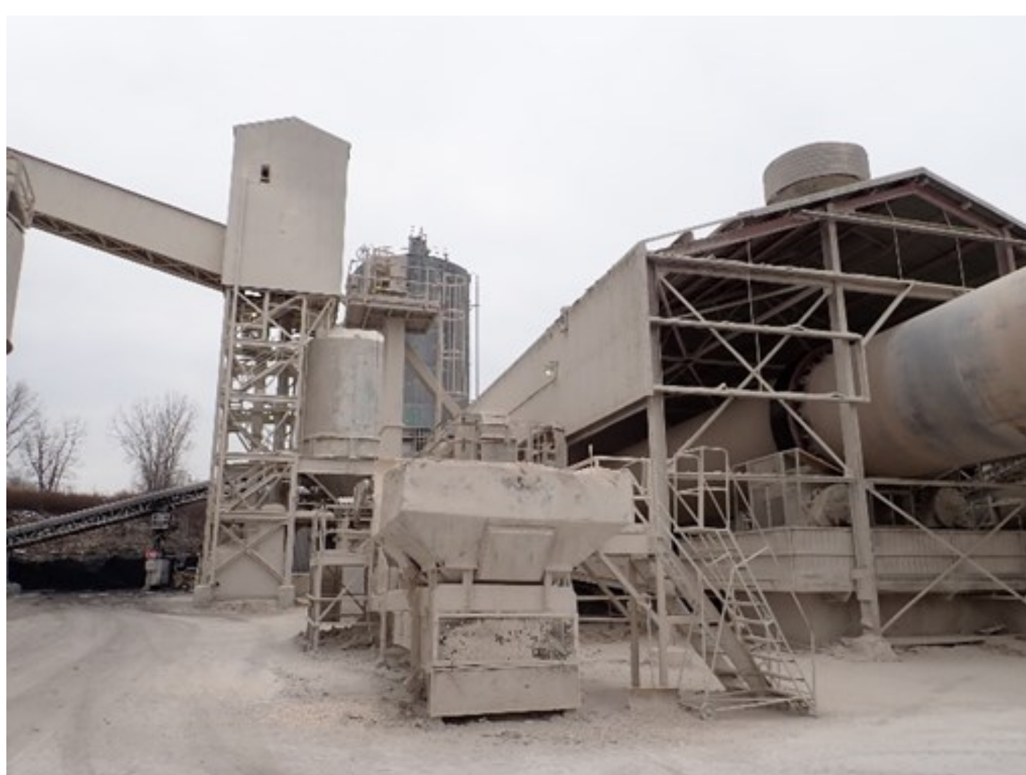
December 2018 - Buggy Hopper and Conveyor
