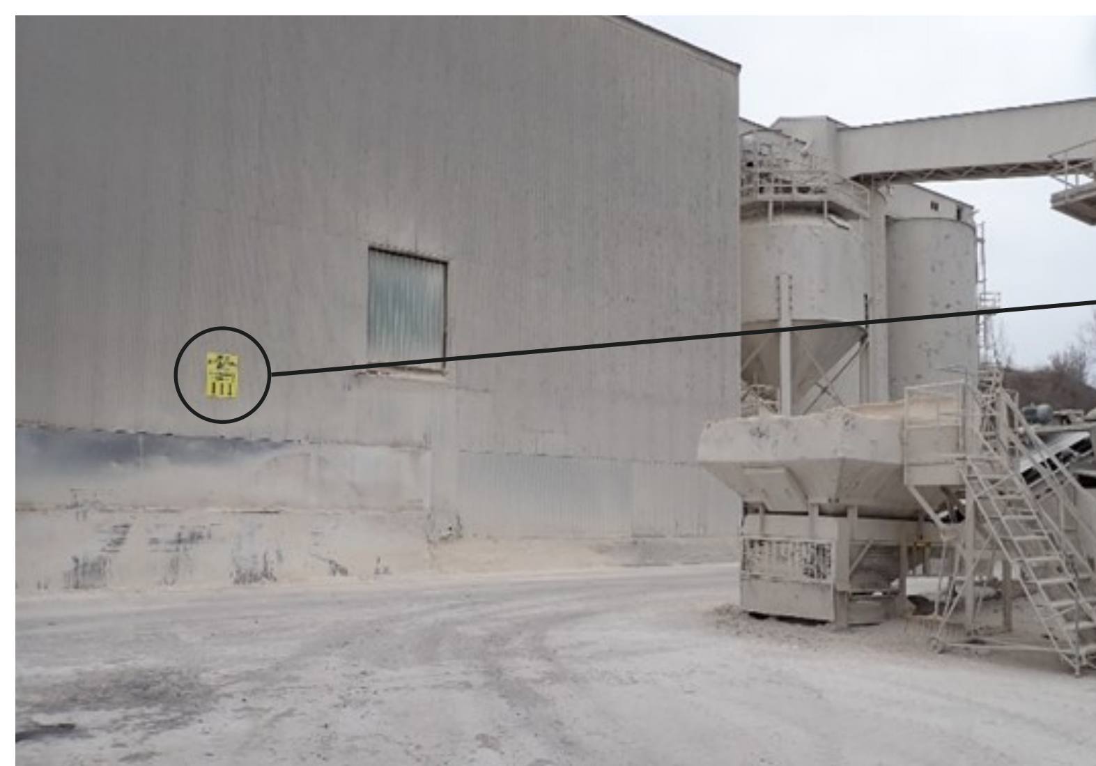
December 2018 - Designated Area for Overloads
