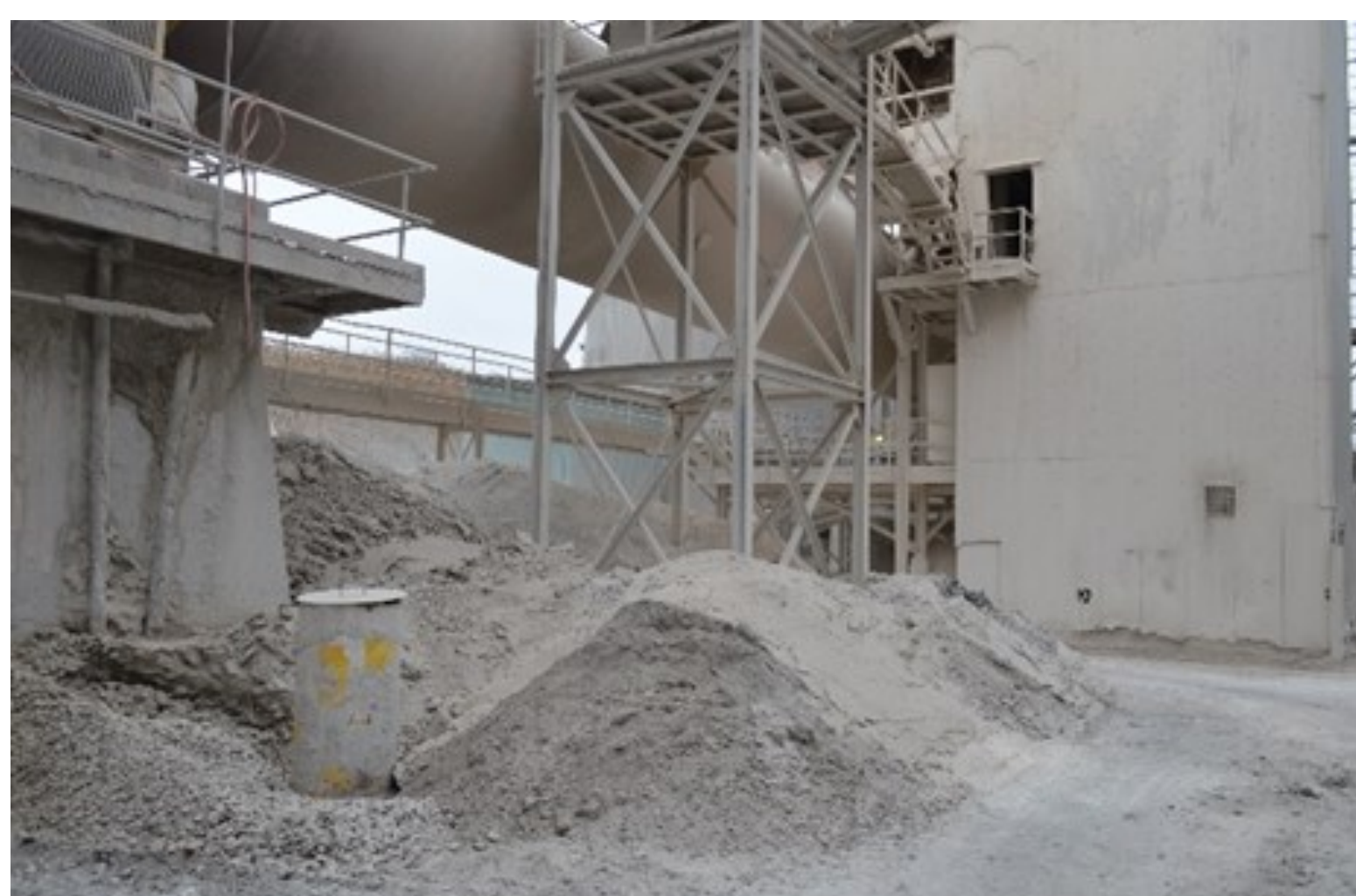
December 2015: Accumulated material in production area and gravel surface
