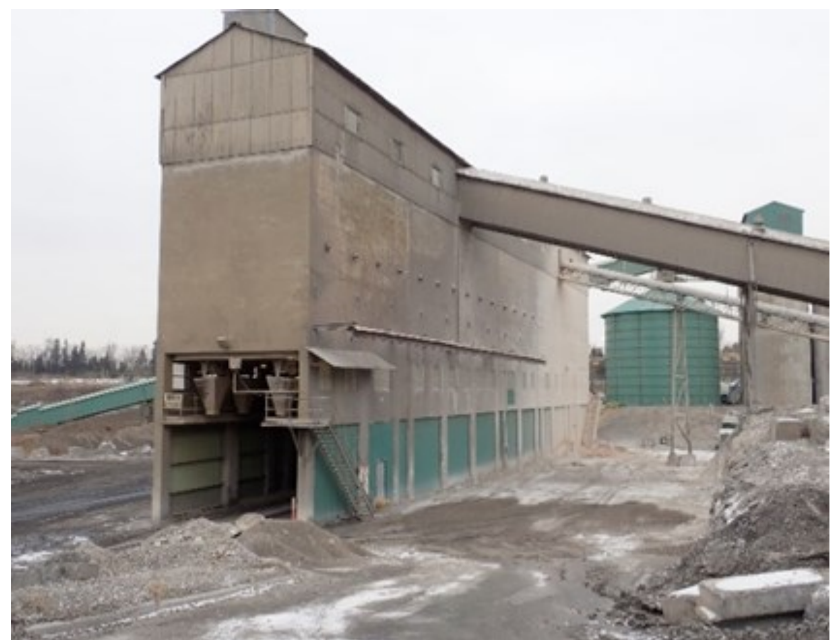
December 2018: Bunker Loadout area enclosed with metal sheeting and pile of lime removed
