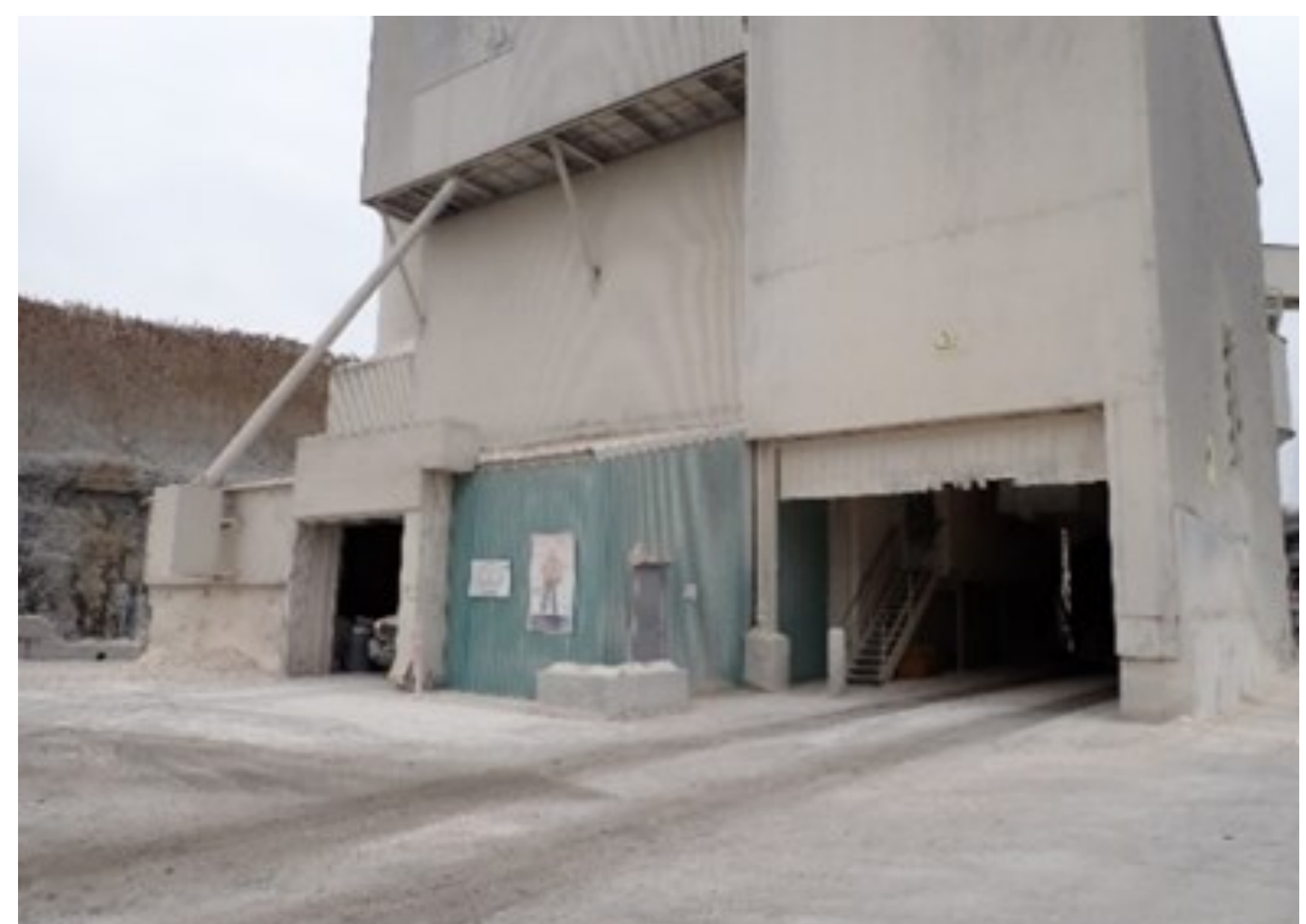
December 2018: Storage piles of lime removed
