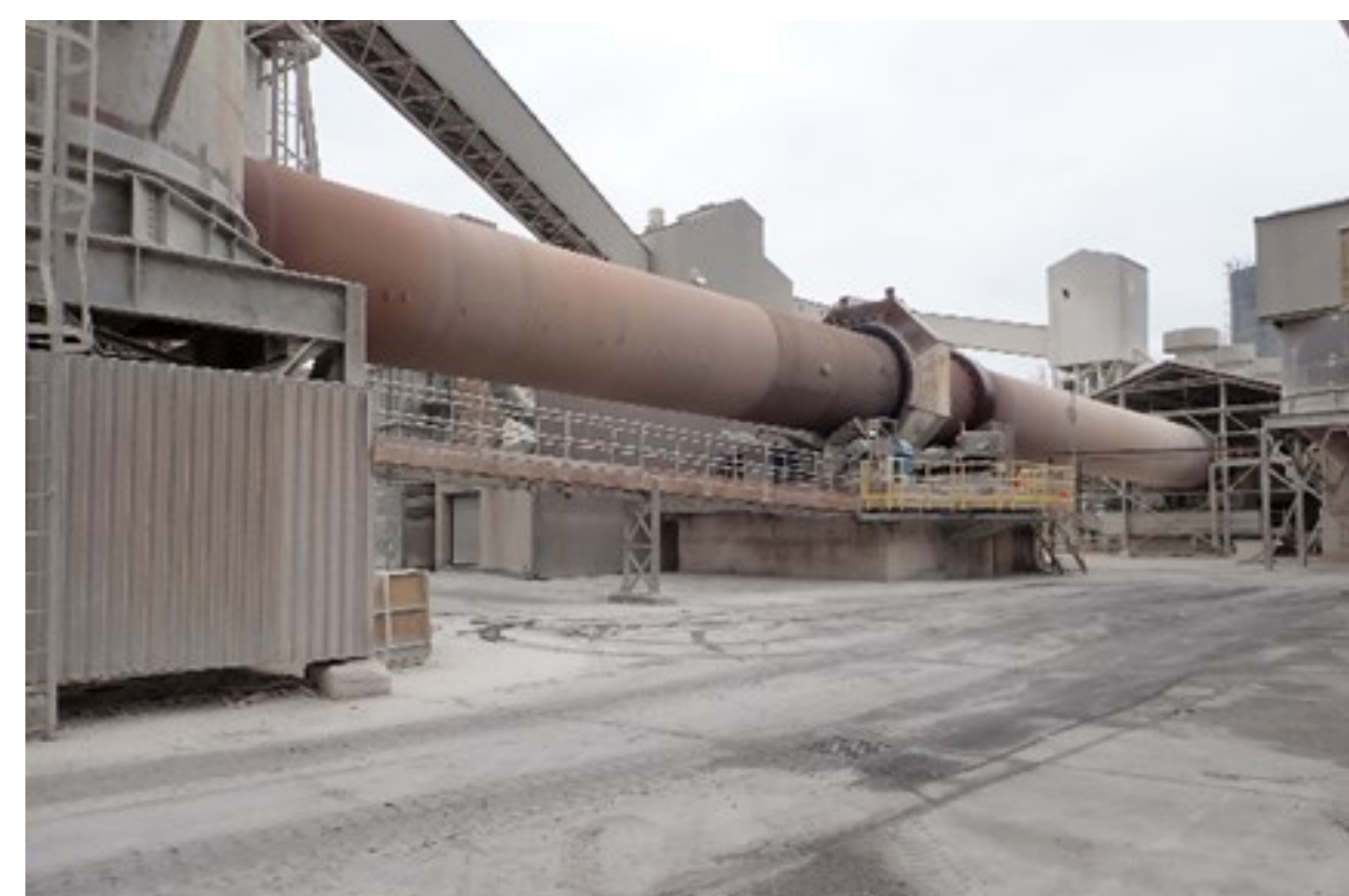
December 2018: Removal of accumulated material and new concrete and pavement
