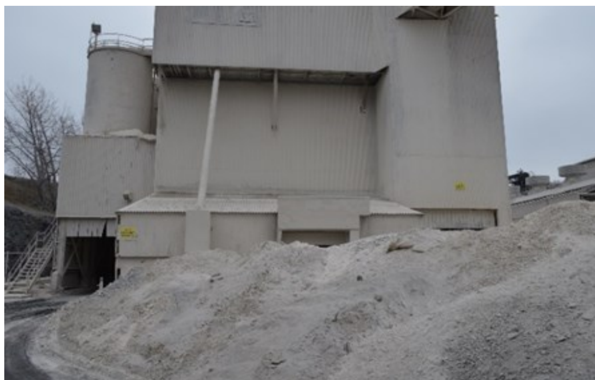
December 2015: Long-term storage of lime in various locations
