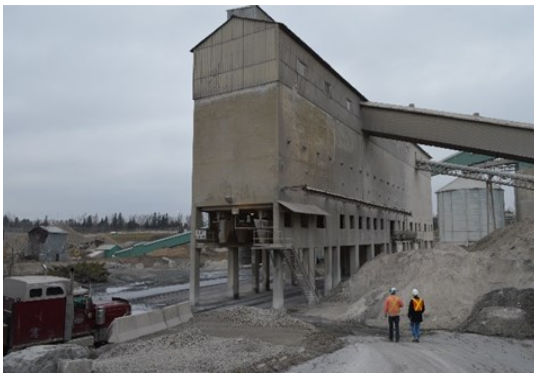
December 2015: Bunker Loadout area open and pile of lime
