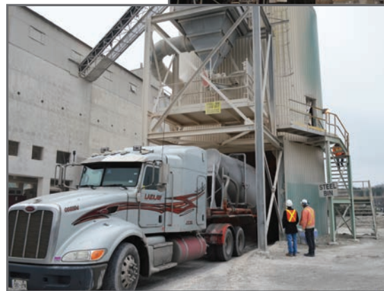
Steel Bin Loadout
