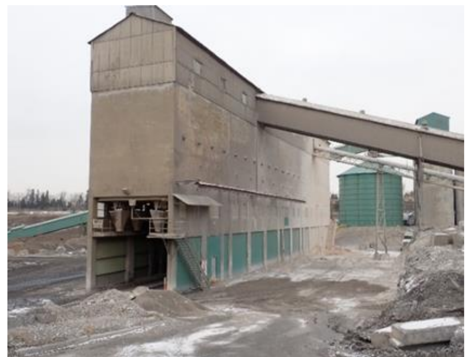
December 2018: Bunker Loadout area enclosed with metal sheeting and pile of lime removed
