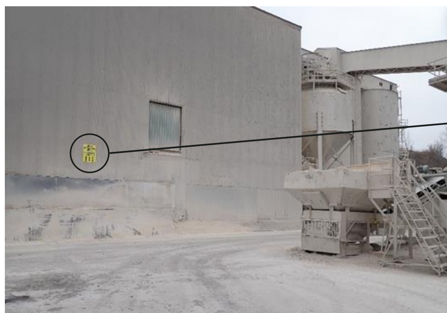
December 2018 - Designated Area for Overloads
