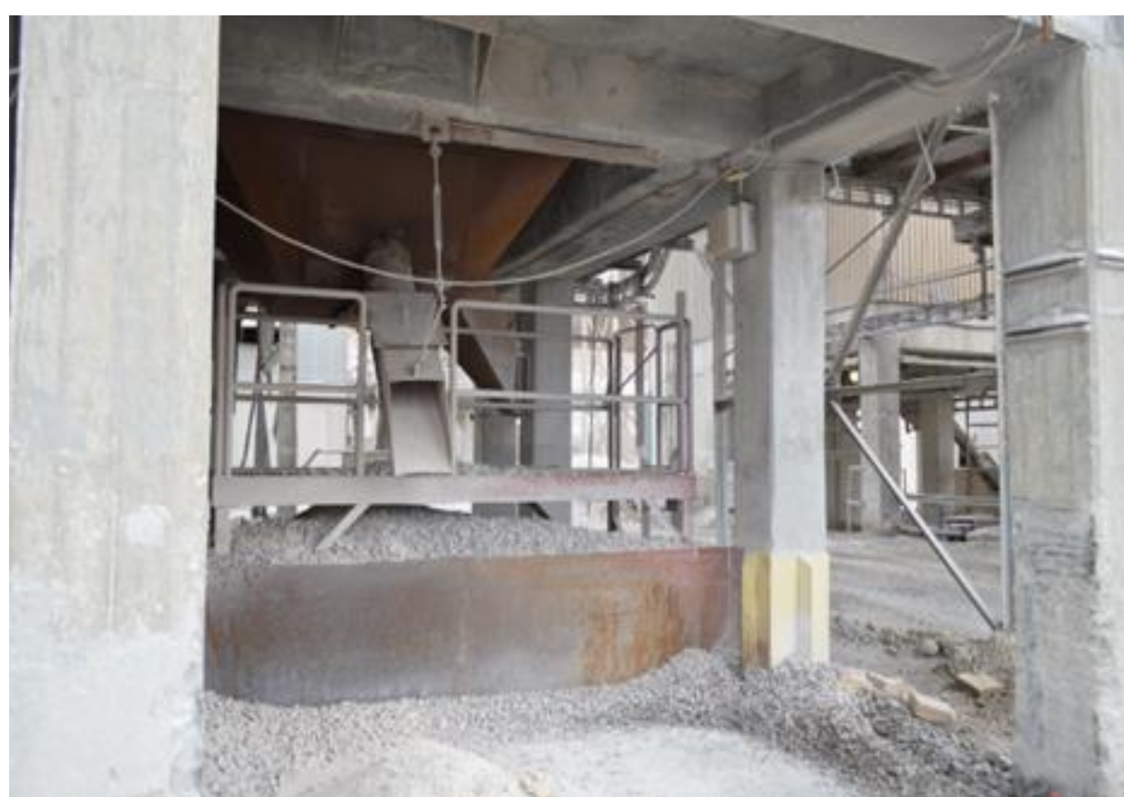
December 2015: Kiln #2 Smoke Chamber Fallout area open
