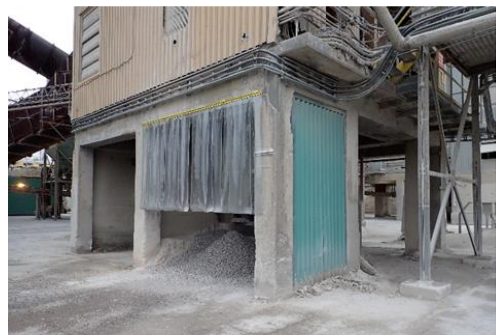
December 2018: Kiln #2 Smoke Chamber Fallout area enclosed with metal sheeting and plastic dust curtain screen
