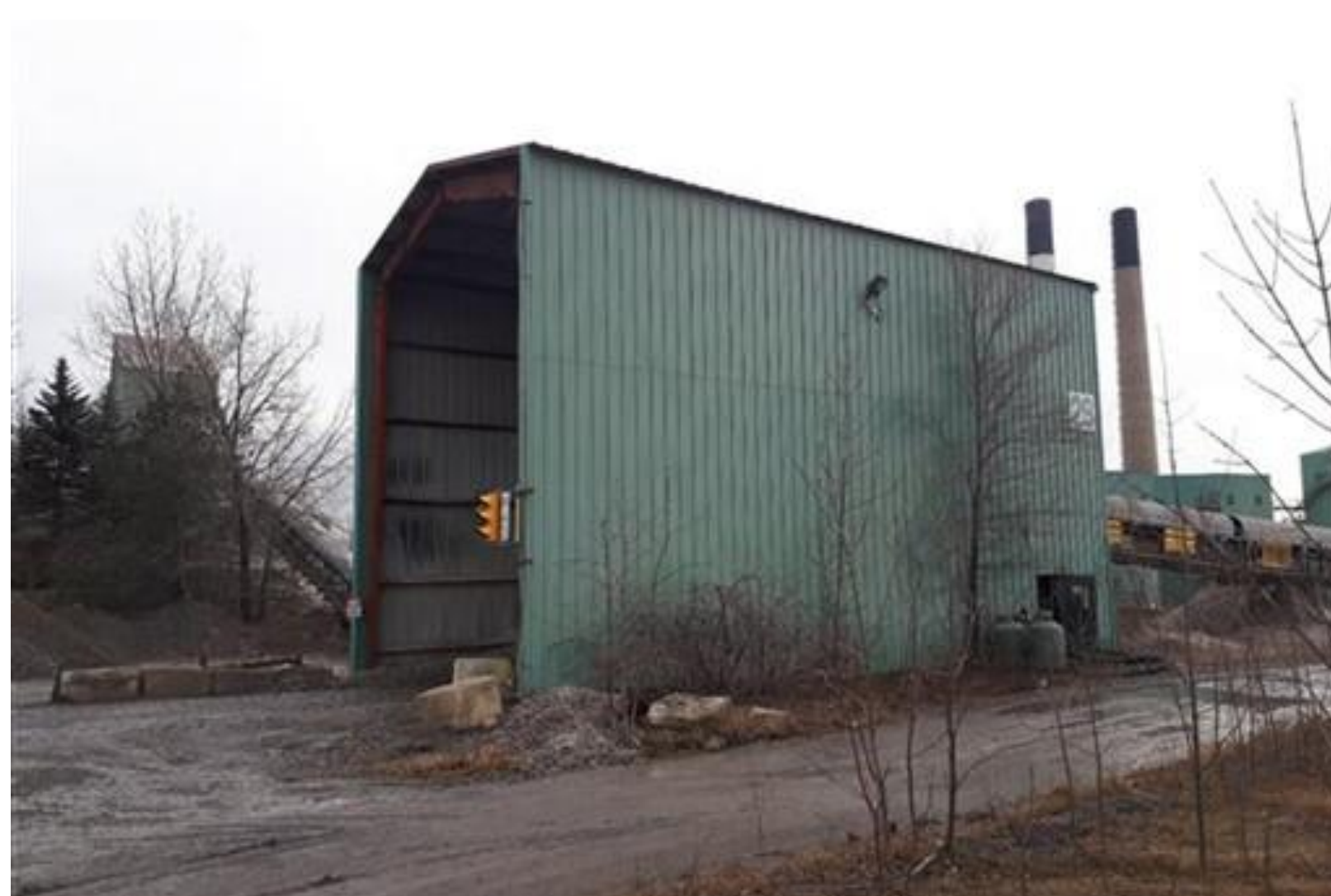
December 2018: Stone Intake Building
