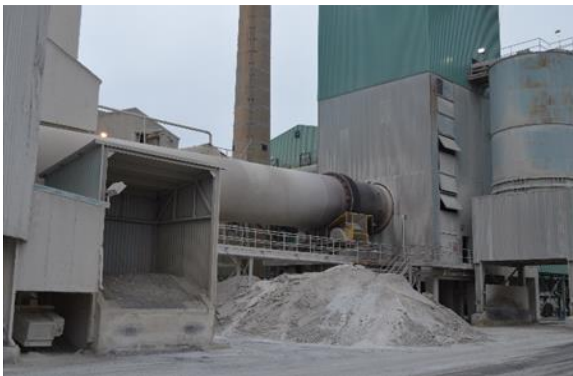
December 2015: Long-term storage of lime in various locations
