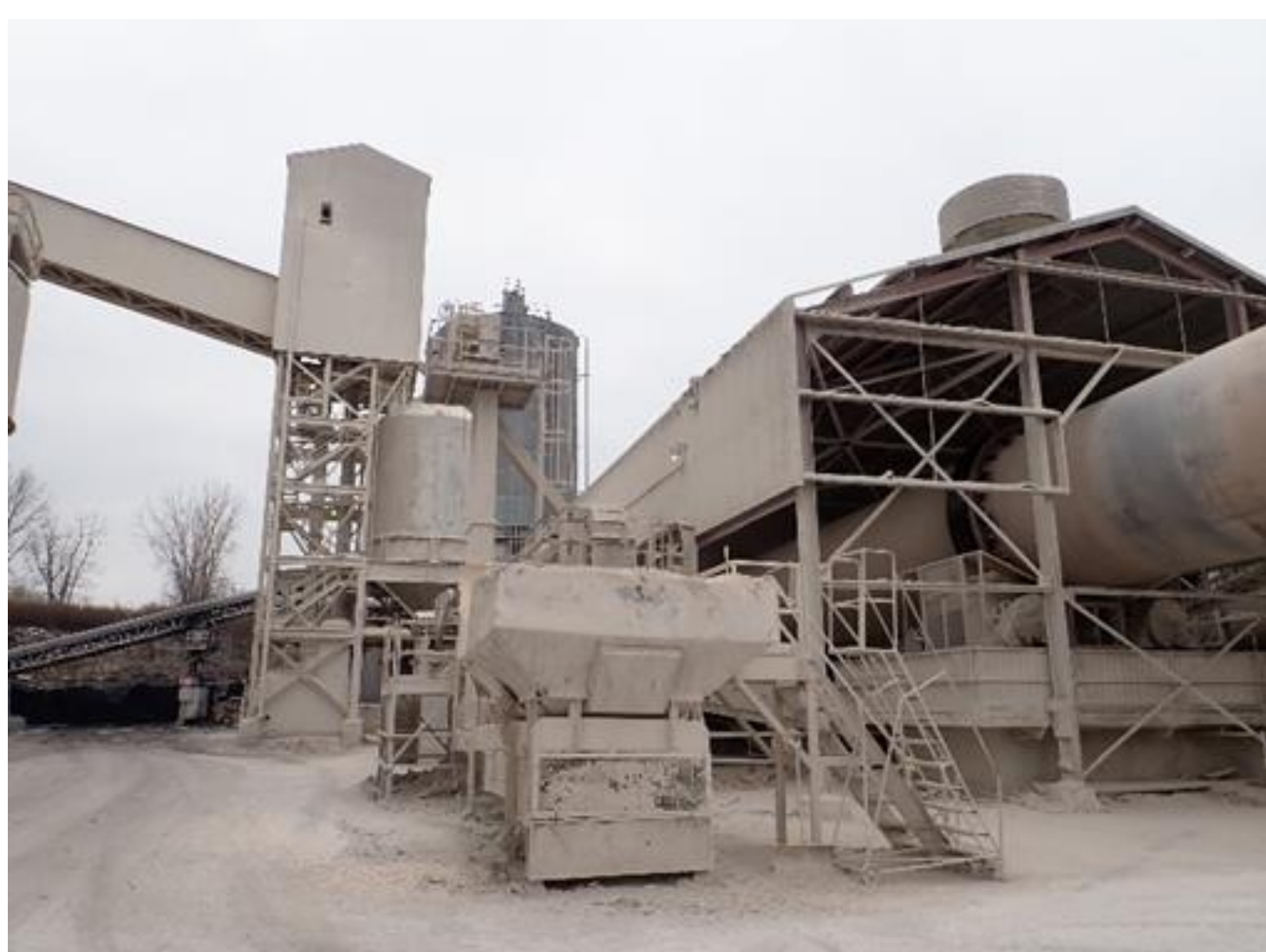
December 2018 - Buggy Hopper and Conveyor
