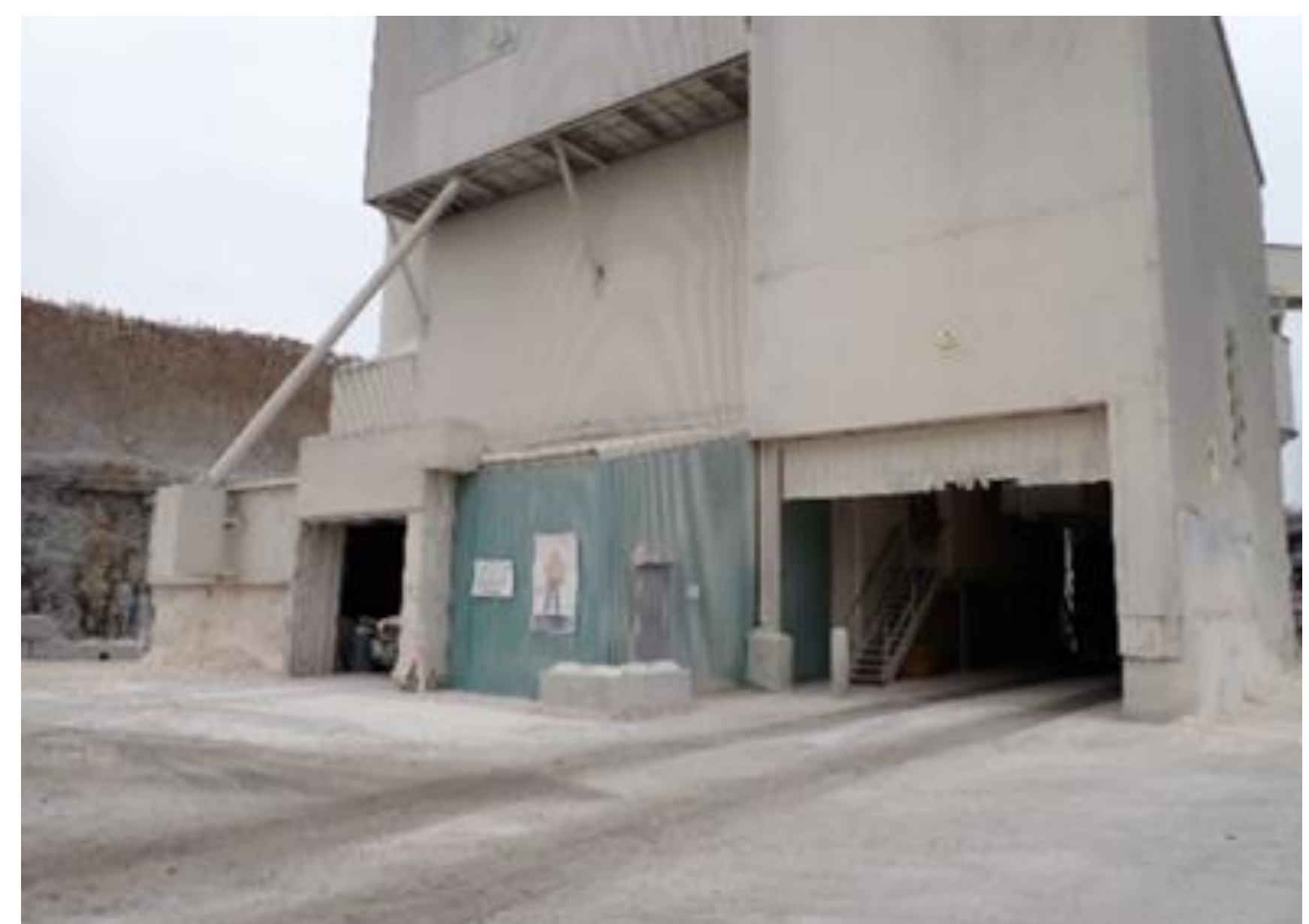
December 2018: Storage piles of lime removed
