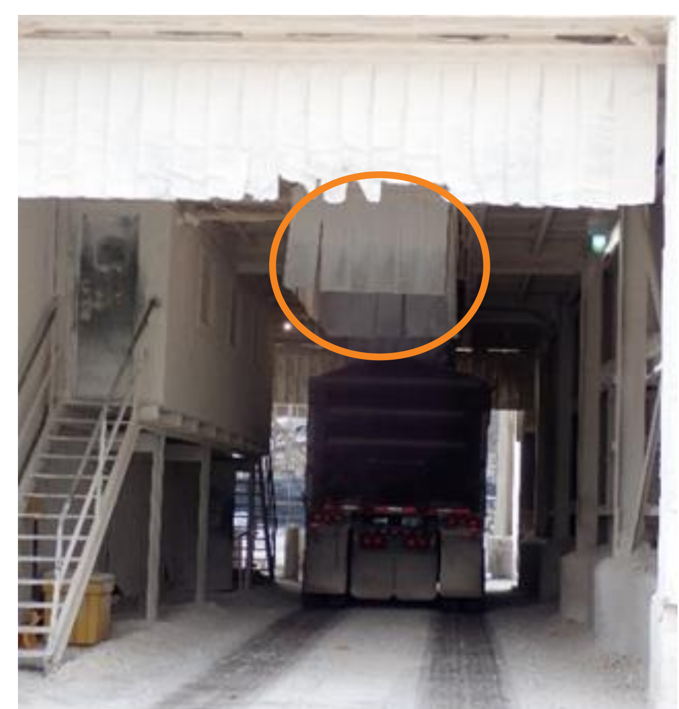
December 2018: Bin 12/13 Loadout area with replaced dust curtains (plastic strips)
