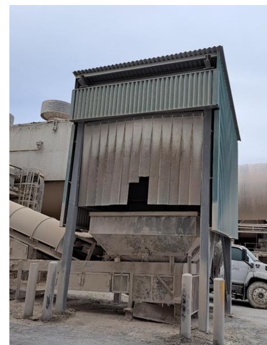
December 2022: Buggy Hopper and conveyor enclosure installed
